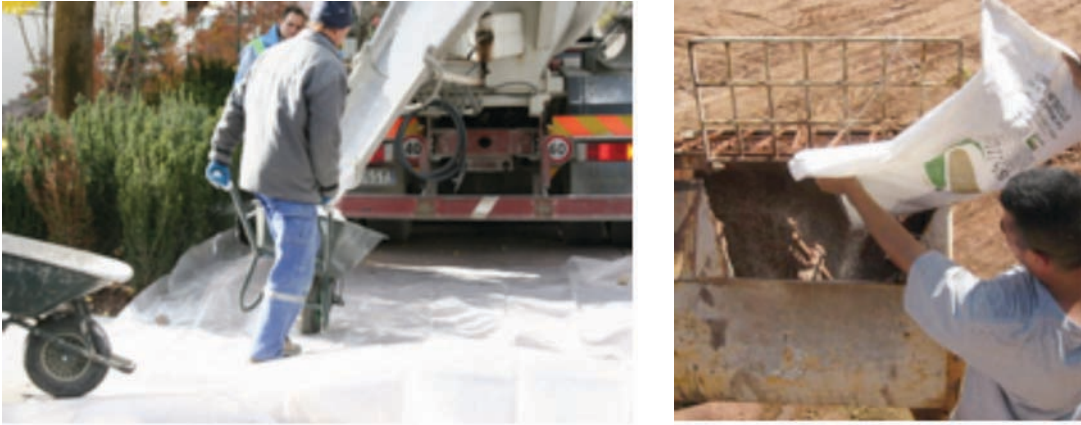
Stabilizer and aggregate blended in two different sized cement mixers
