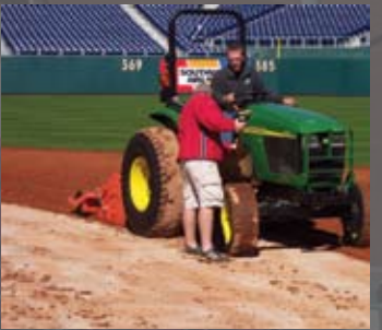
Photo: Stabilizer installation at Citizens Bank Park
